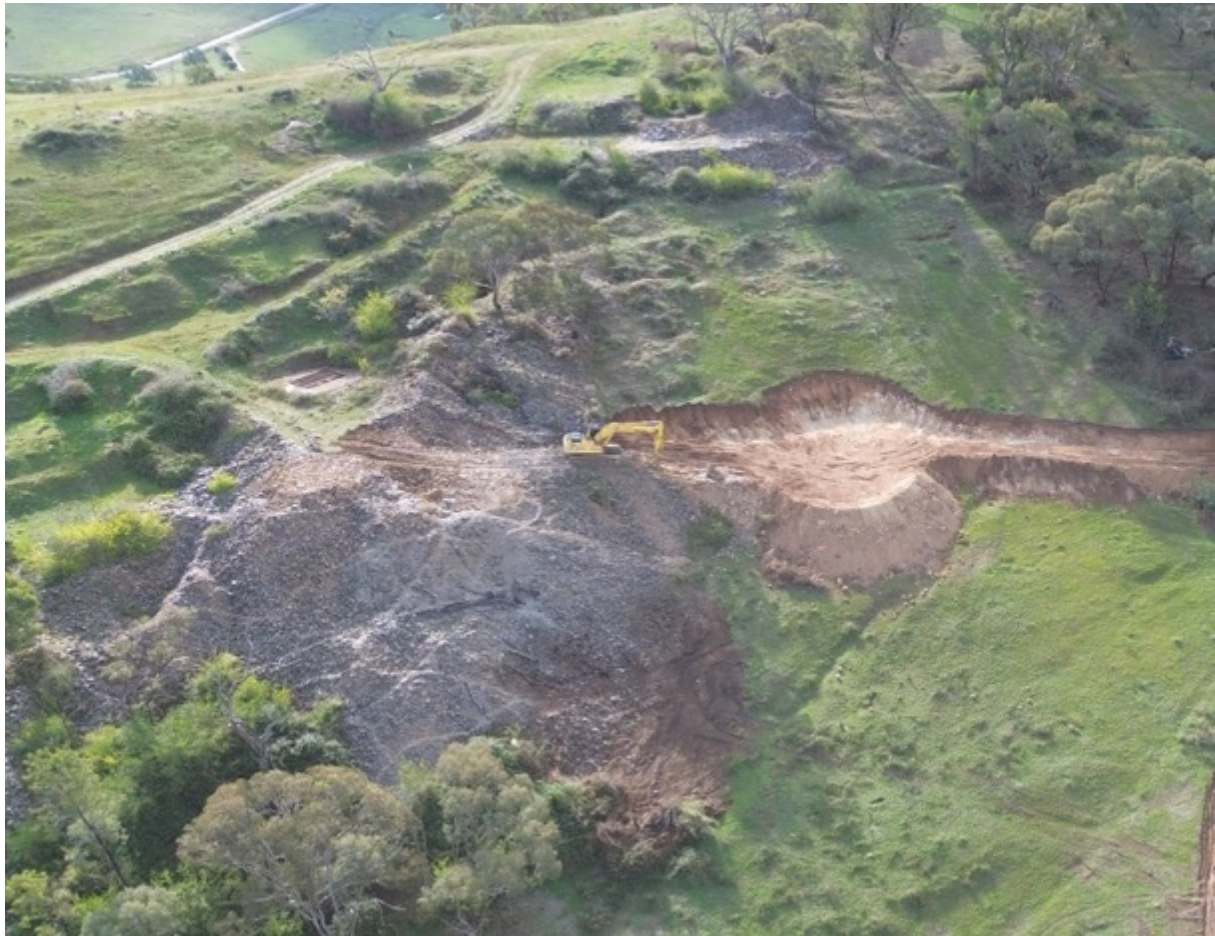
Mineralised waste recovery has commenced at Challenger
